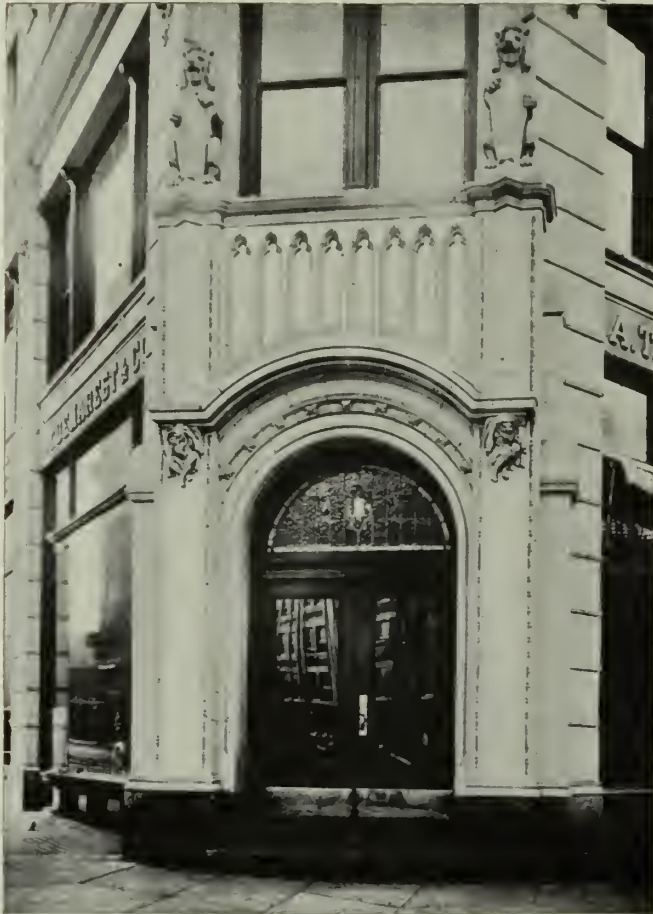
MAIN ENTRANCE TO DEMAREST BUILDING, NEW YORK CITY. Executed in cream white terra cotta by New York Architectural Terra Cotta Company. F. H. Kimball, Architect.
